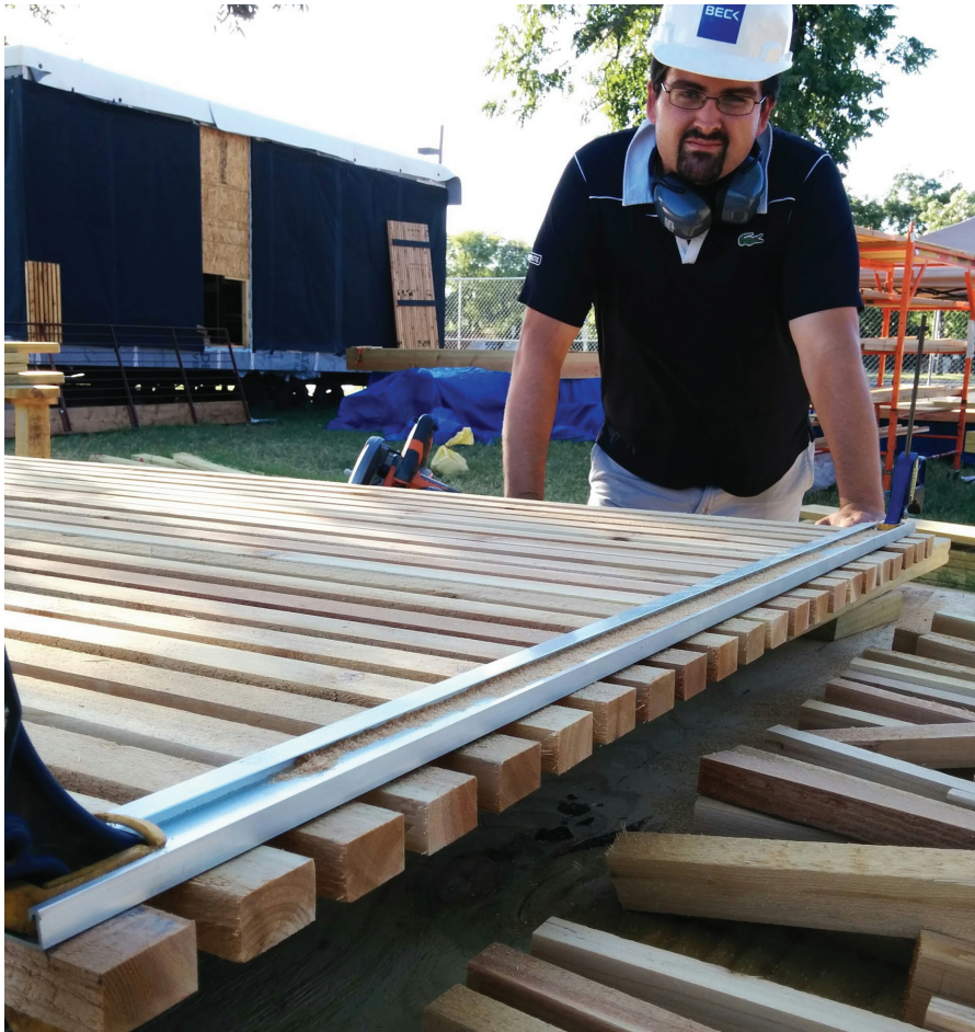
Fig. 02 Final cut of the bottom of the rainscreen insuring the exact length of each individual piece.
