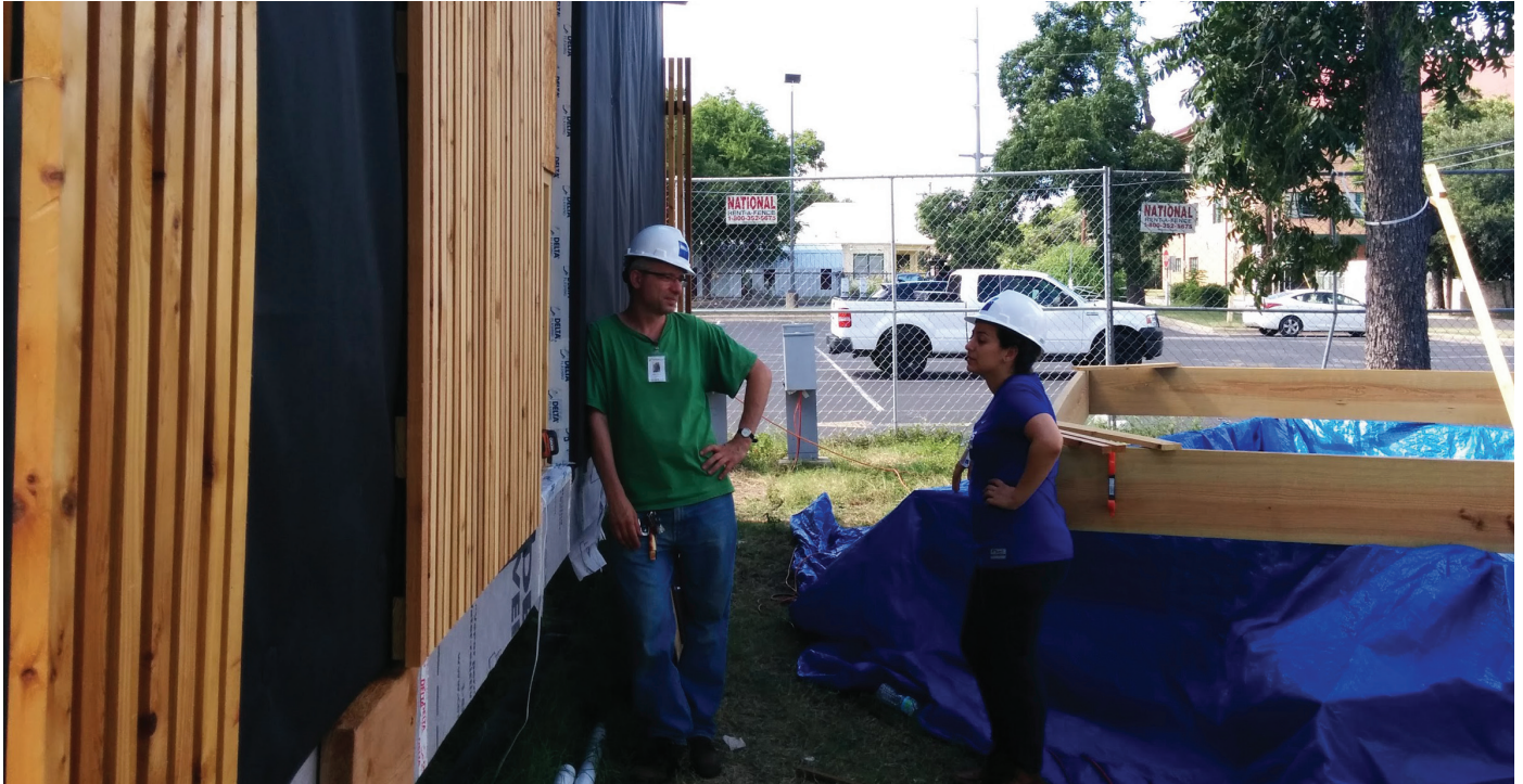
Fig. 03 Team discussing the installation of rainscreen panel on exterior wall.
