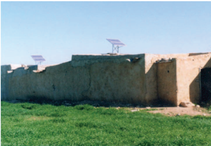
Figure 3 - Photovoltaic kits were provided to remote villages to electrify region that were too far away from the grid. (ONE)
