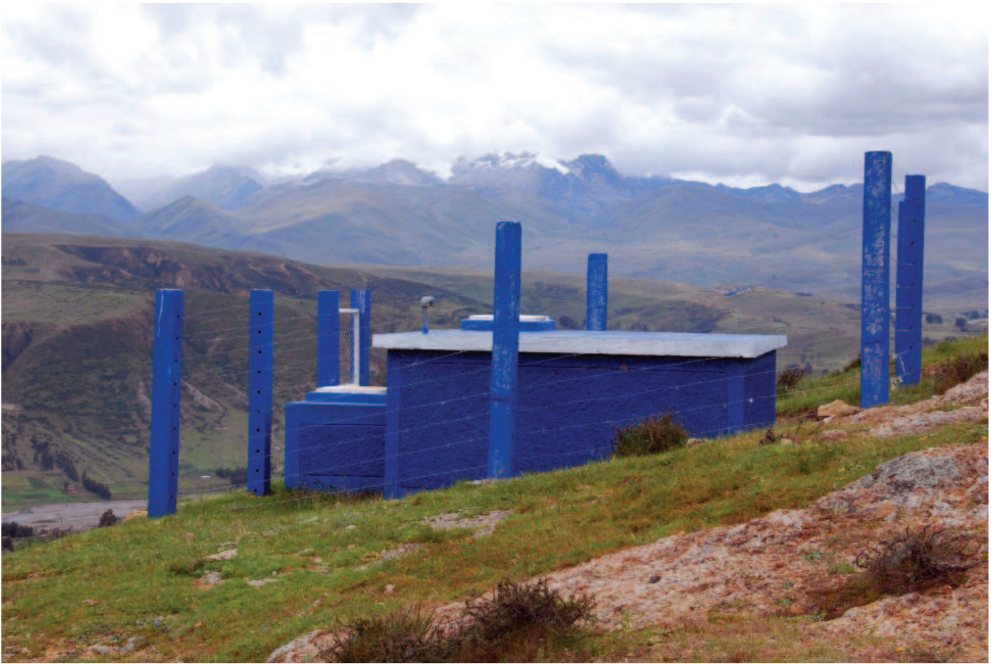
Figure 2: Water storage tank above Yanamito village at about 3800 m. (courtesy of Daene McKinney)
