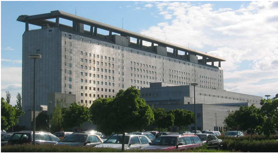
Fig. 06 Exterior view of Klinikum Großhadern from the grounds of the hospital. Klinikum Großhadern is the fourth largest hospital in Germany and the largest in Munich. The building features aluminum panels used to reduce heating and cooling loads. The building looks metallic and is known as the "toaster" by the attending medical students.
