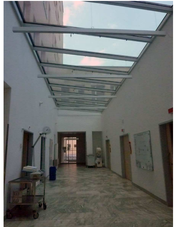
Fig. 23 Emergency rooms have a sky light in their main corridor
