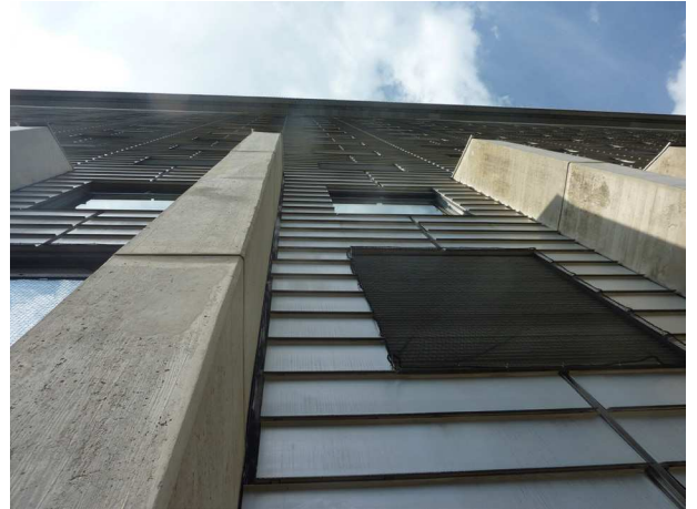
Fig. 08 Interior courtyards are surrounded by large building facades making them uncomfortable to be in.
