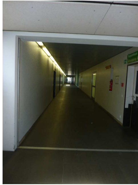
Fig. 14 Poorly lit halls
